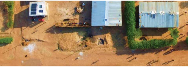
FIG 8 SolarworX project Cameroon is redefining energy access in the remote regions of West Central Africa.
